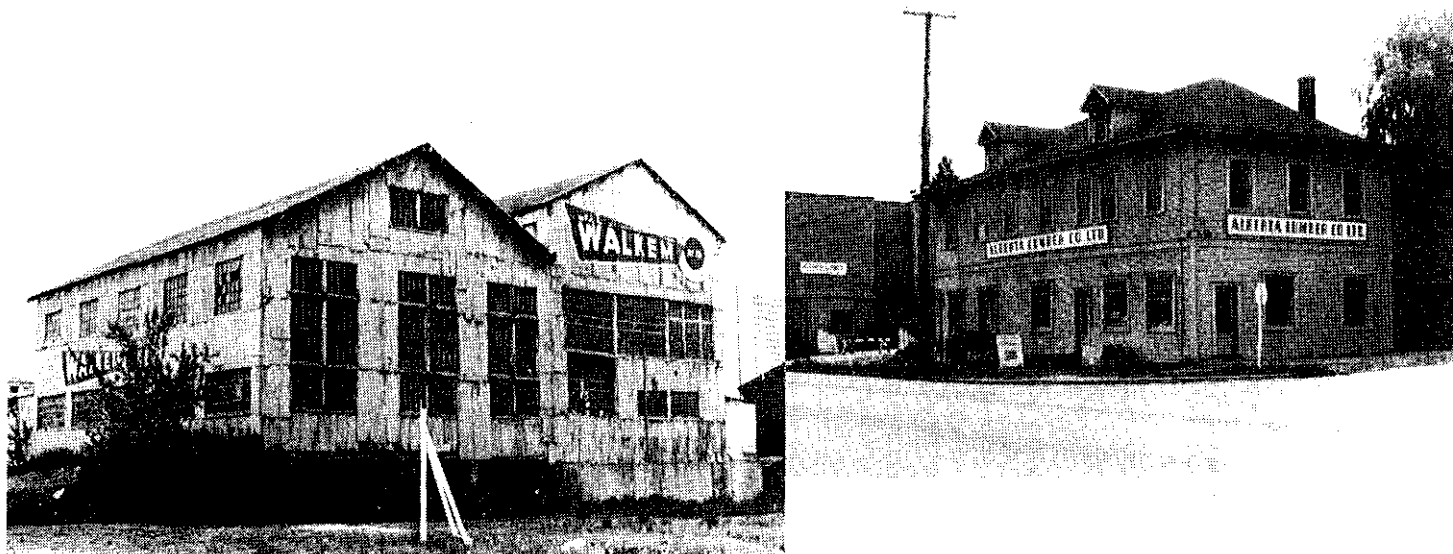
Walkem Machinery , once just west of the south end of the Cambie Street bridge, was a classic in corrugated metal. Note weathering, broken panes of glass.
